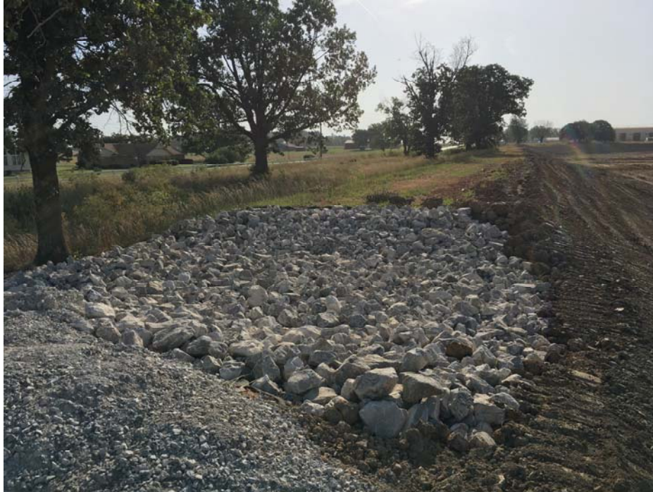
Photo 7 – Emergency Spillway with Riprap lining
