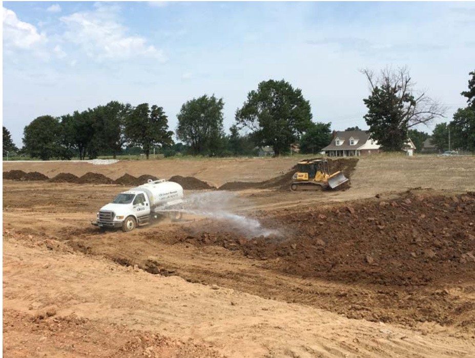
Photo 1 – Watering and Placing Clay liner in Sedimentation Pond
