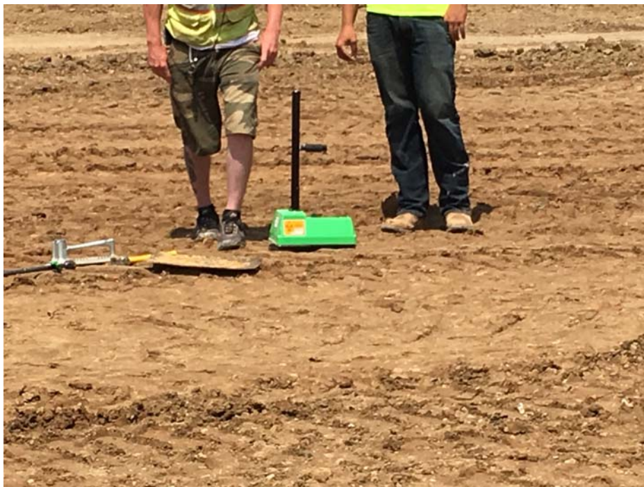
Photo 2 – Density Testing Clay Liner
