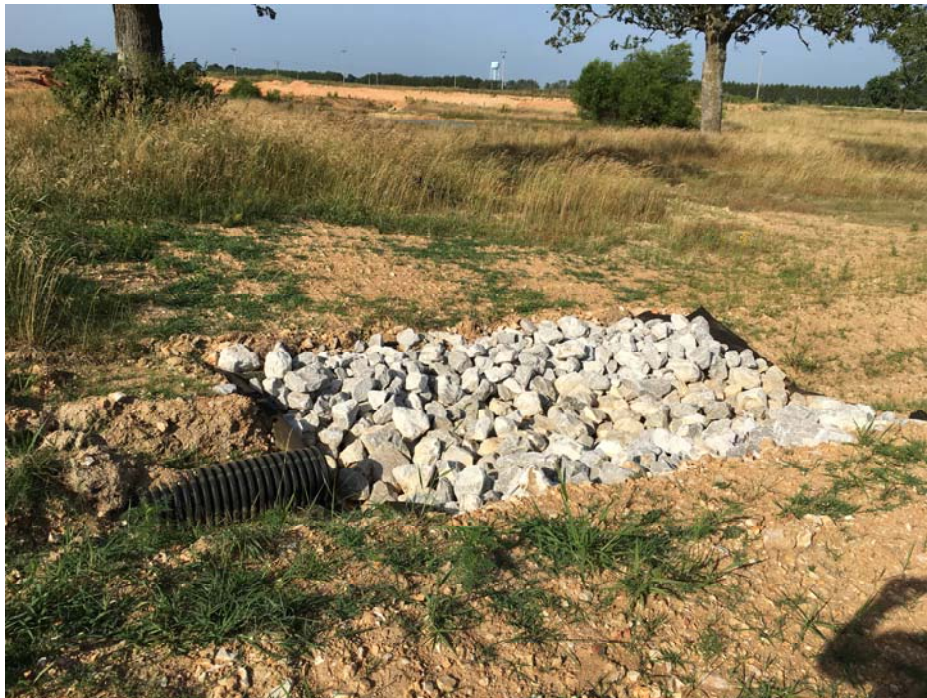
Photo 8 – Outfall Pipe with RipRap apron
