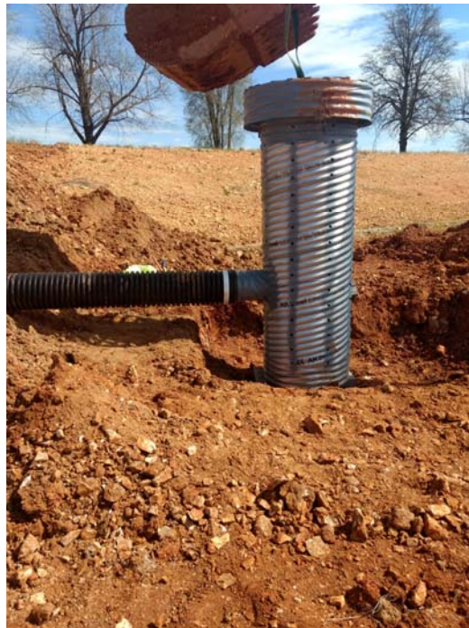
Photo 4 – Principle Spillway connected to discharge pipe
