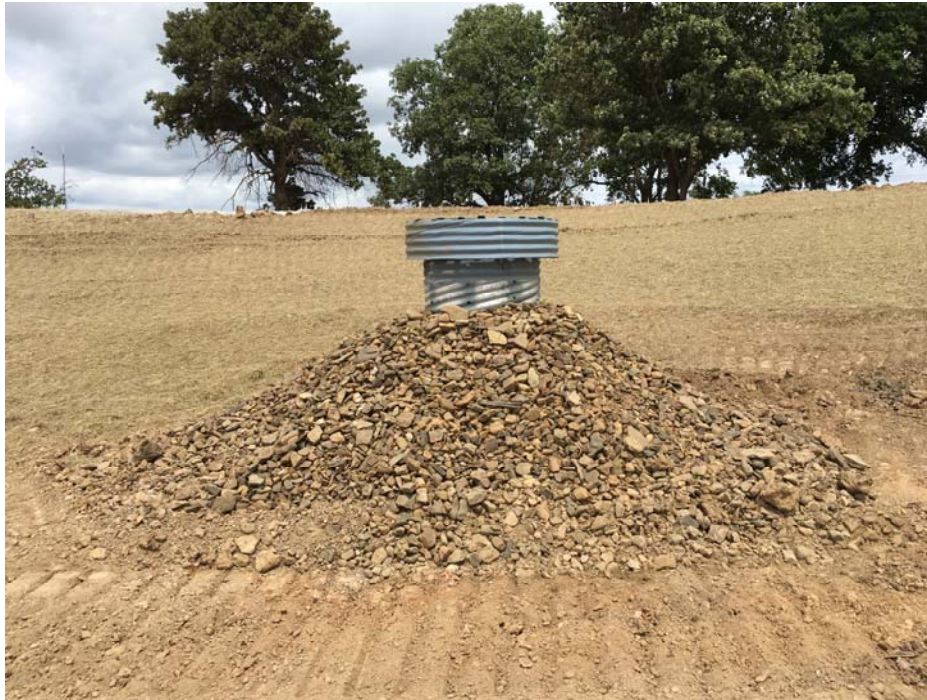
Photo 5 – Principle Spillway
