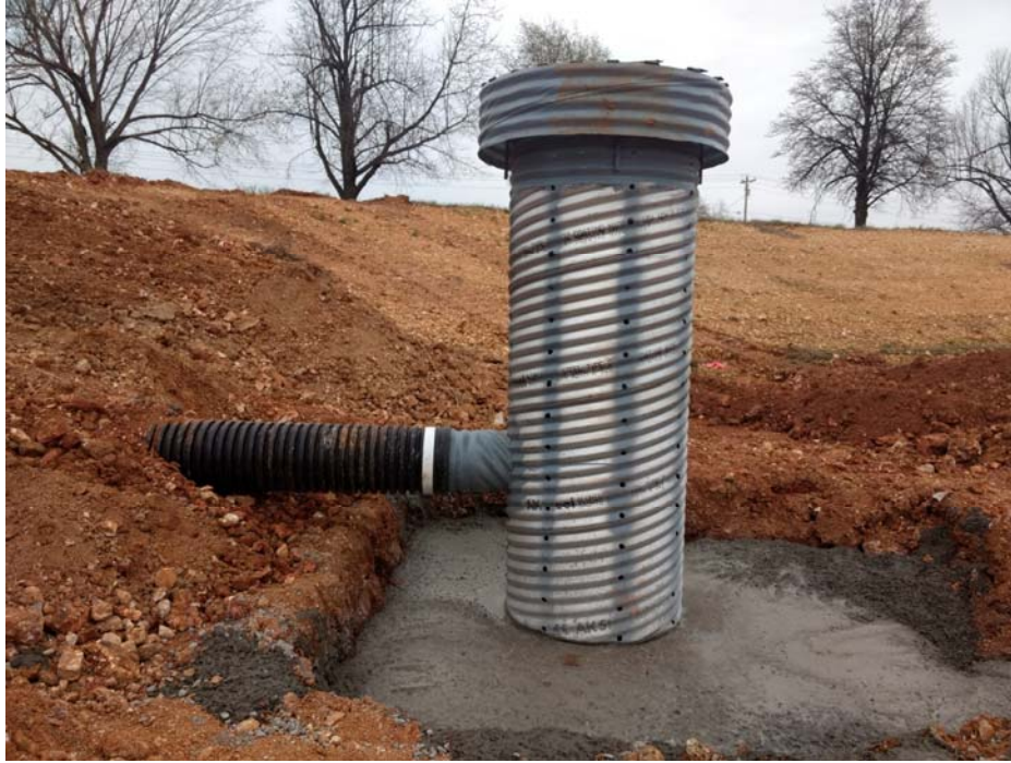
Photo 3 – Principle Spillway: 36" Riser Pipe
