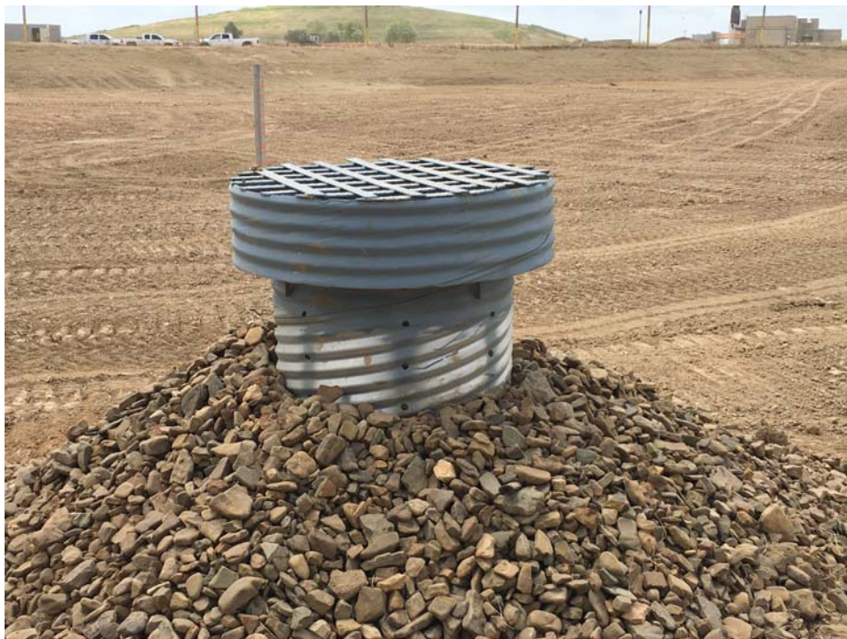
Photo 6 – Principle Spillway: 36" riser with trash rack
