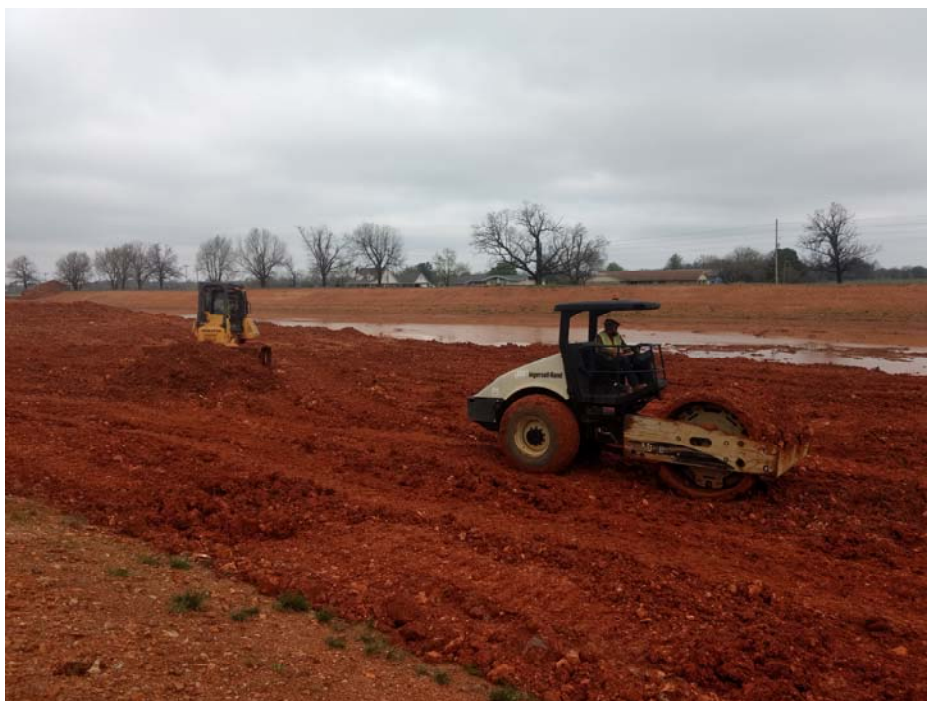
Photo 12 – Placing and compacting Scalehouse pad
